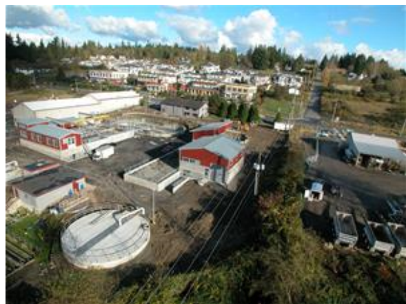
Figure CF-1. Duvall Wastewater Treatment Plant Source: City of Duvall
