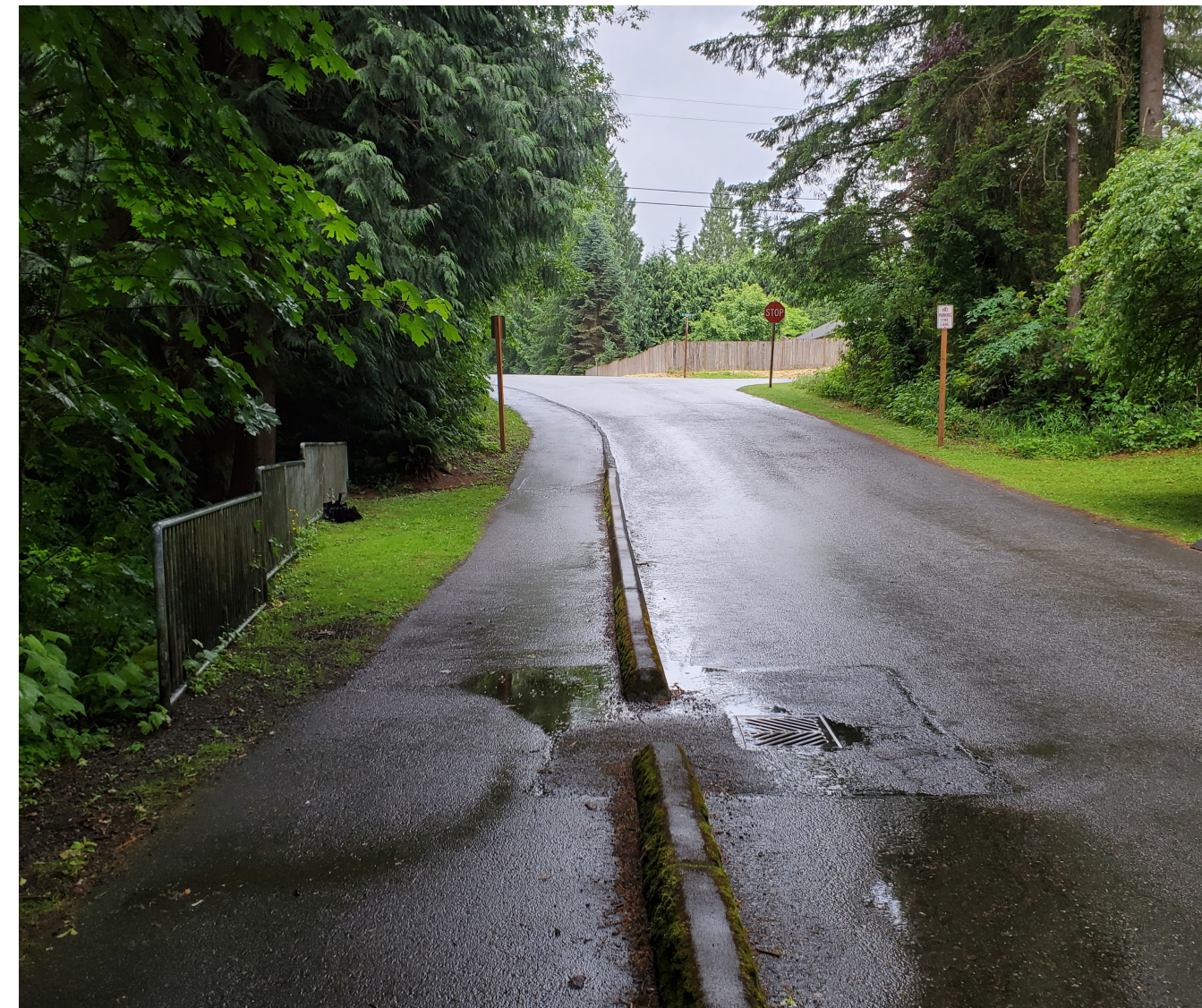
Existing Stormwater at Coe-Clemons Creek Crossing, Duvall
