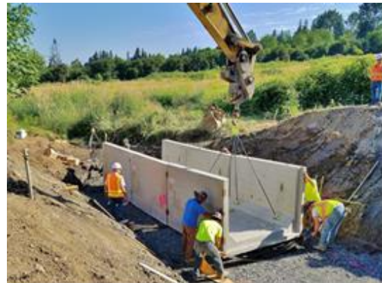
Crews Install Culvert Sections at Thayer Creek
