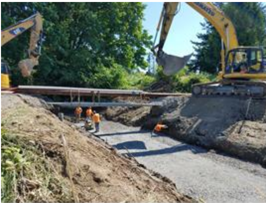
Crews Excavate Roadway on NE 143 rd PI Preparing for Culvert
