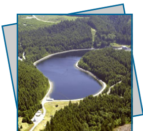
The Regulating Basin, photo courtesy of Seattle Public Utilities: Water from the Tolt Dam enters the Regulating Basin where it is stored before entering the transmission line.
